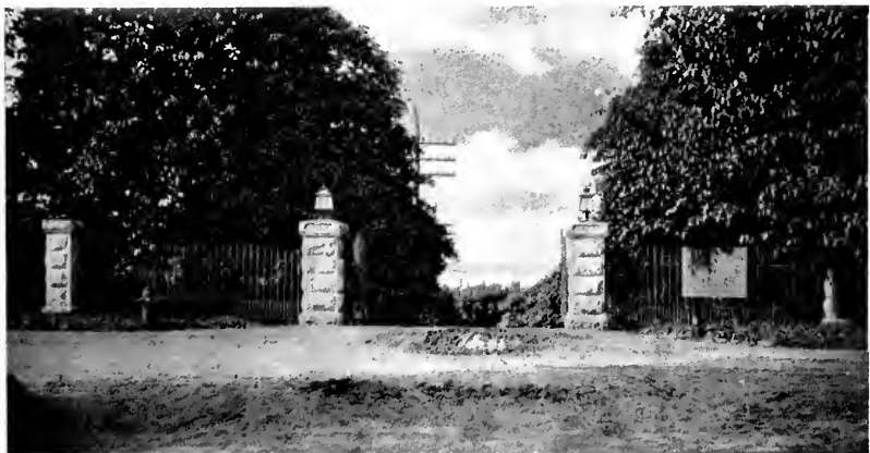
THE MARGARET GATE ENTRANCE TO BAY CREST, HUNTINGTON, LONG ISLAND
